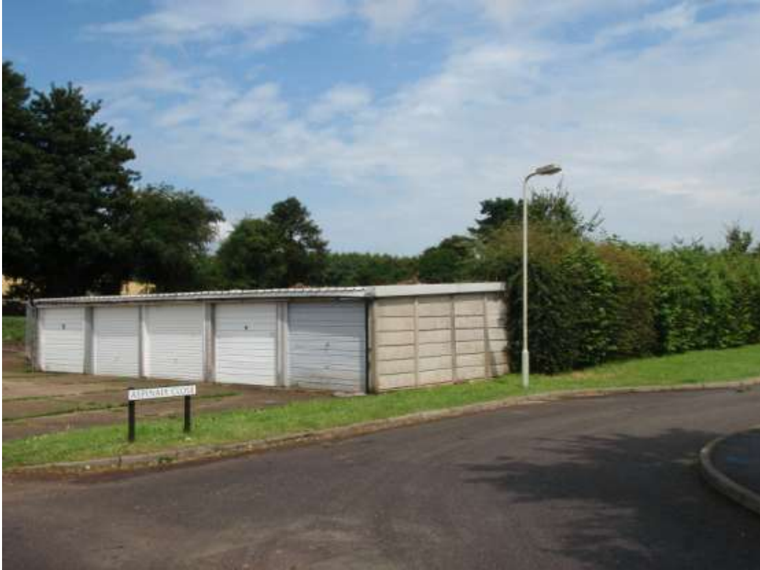
Plate 3. View of site from top of Cranmer Close (looking north)
